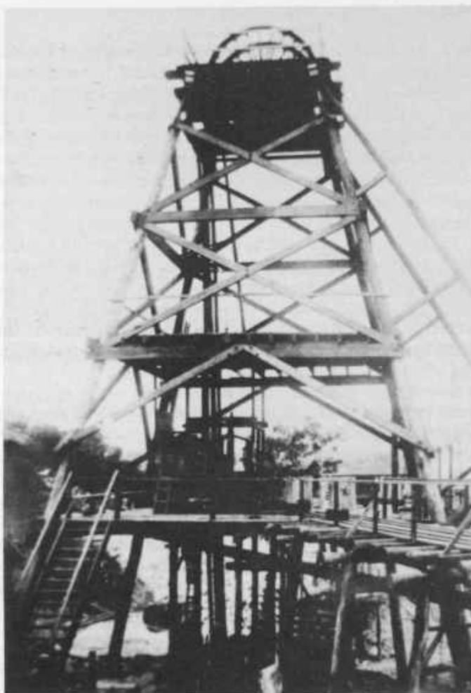
New pithead gear built around an existing poppet head, Kennedy shaft, Mount Perry. Source - Maryborough, Wide Bay and Burnett Historical Society.
