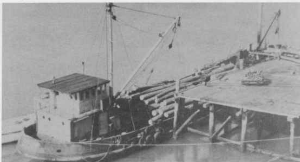
Goori - Wilson Hart's wharf 1958. Note the trolley of firewood on the wharf which is waiting to be loaded onto the vessel. The Goori had no main engines, its boiler was used to power auxiliary machinery. Neil Simpson's collection.
